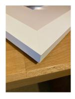
Frames to be finished to a good standard, with no excessive gapping at the mitred corners.
